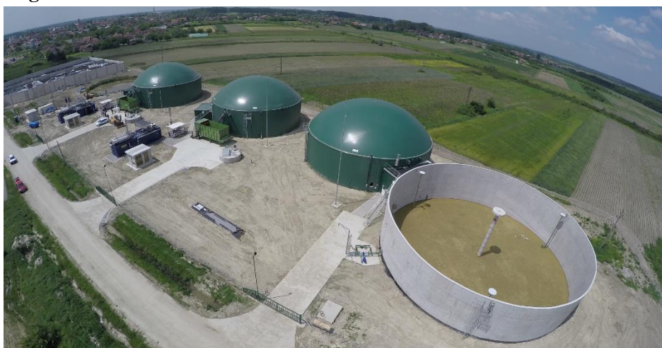
Figure 17 Biogas CHP Plant in Bac: Aerial view onto digesters, feeders, biogas storage, engine containers and transformers
